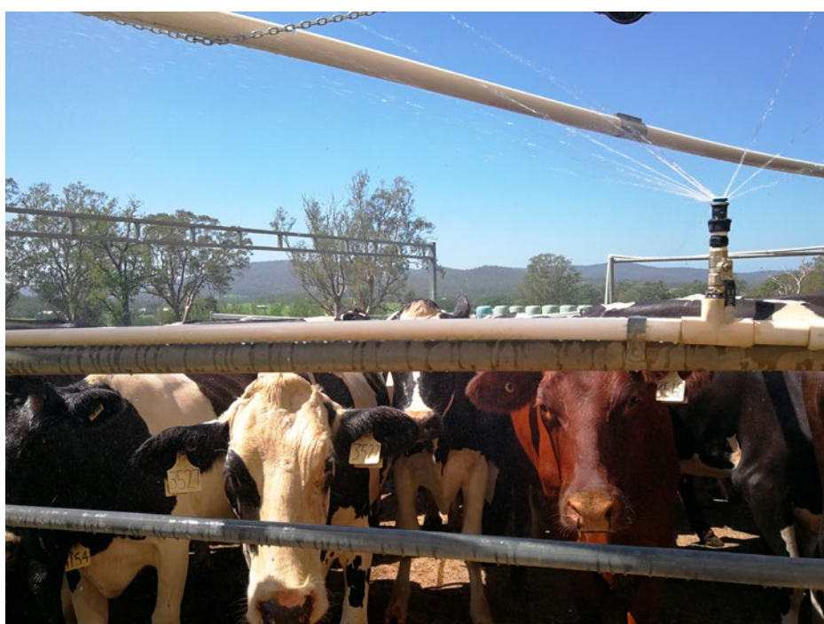
Sprinklers in milking area.
